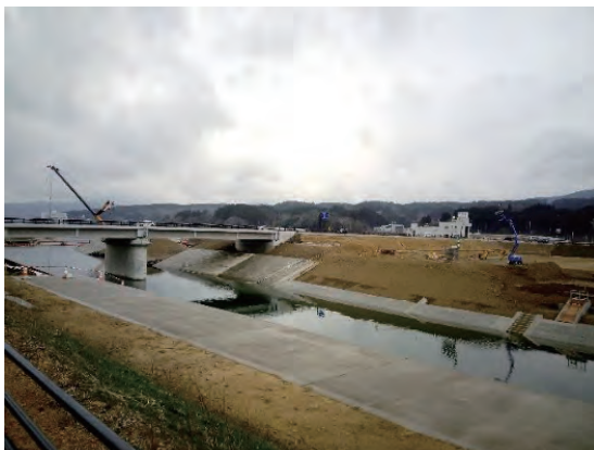
Reconstruction work at Onagawa, March 2019
