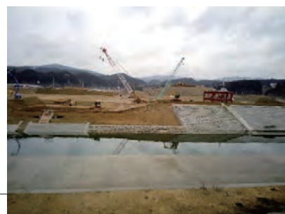
Reconstruction work in Tohoku, March 2019
