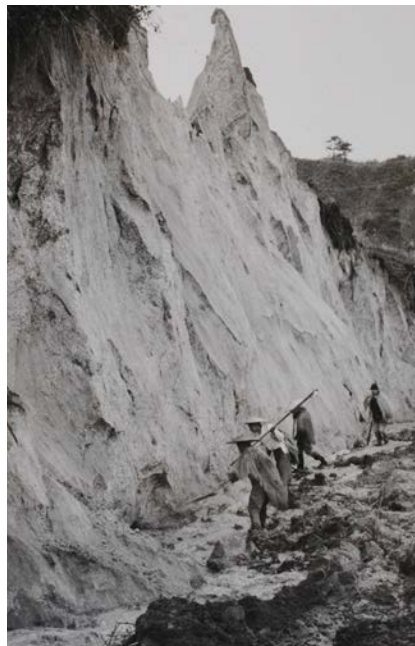
Extracting iron sands in the early 20th Century, Okuizumo ©Hitachi Metals, Ltd
