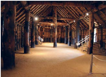
One of the large buildings at Sannai Maruyama has a floor area of 252.4sqm and walls 7.5m high, supported by 19 thick pillars ©Aomori Prefecture
